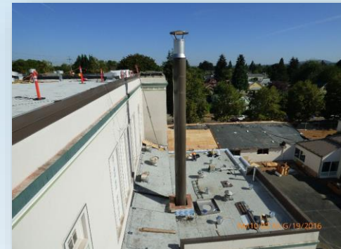
Sellwood MS New Chimney Stack
