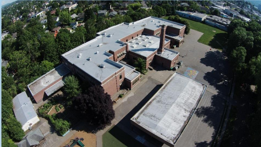
Abernethy 29,000 SF of New Roofing
