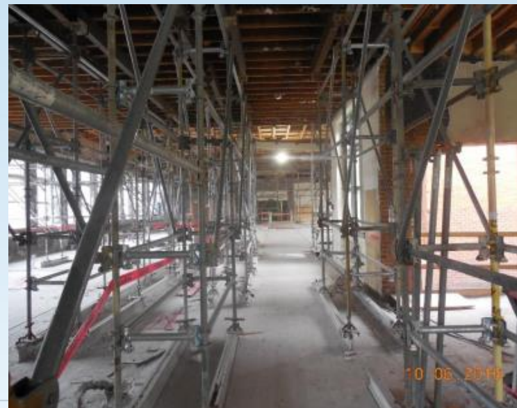
Shoring in Historic Building
