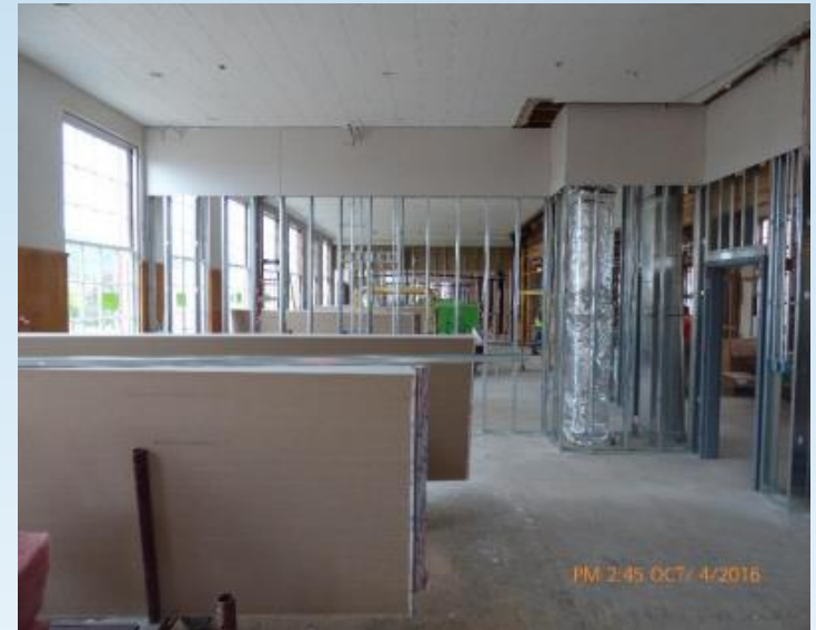
Historic Modernization Interior
