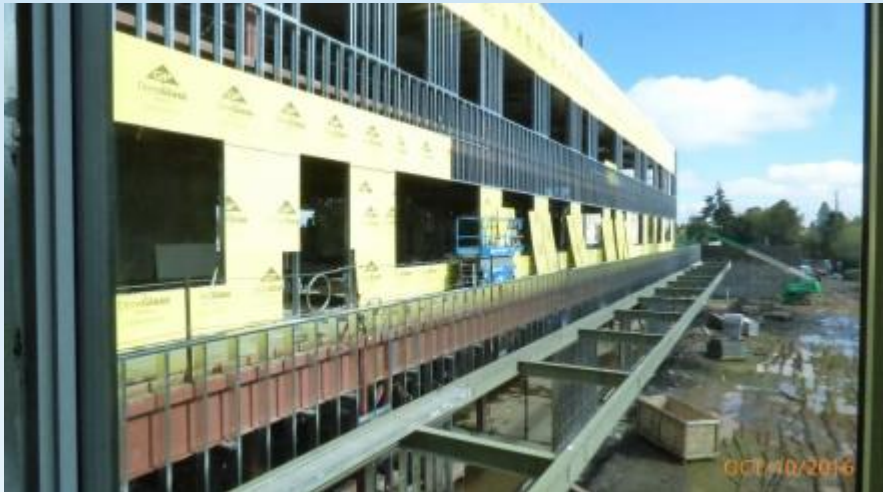
Exterior Walls Ongoing
