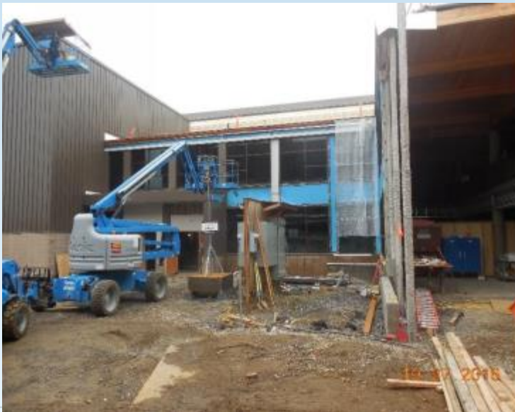
Permanent Drying in of Commons
