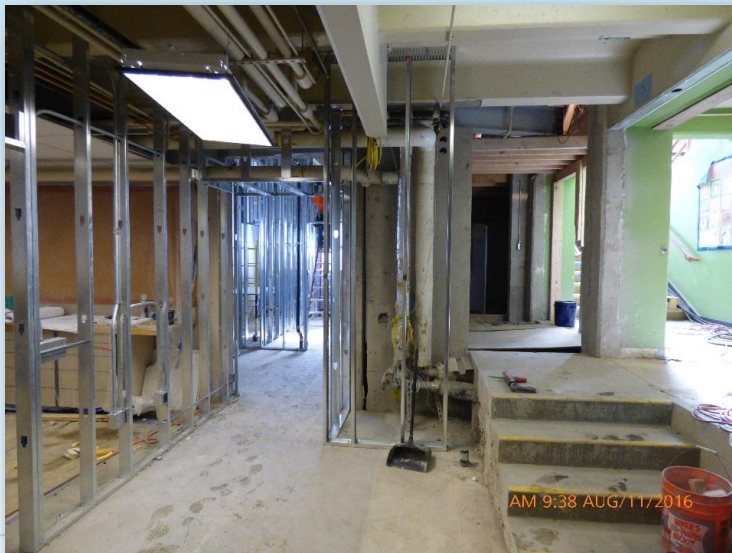
Chavez – During and After Framing Around New Elevator Shaft
