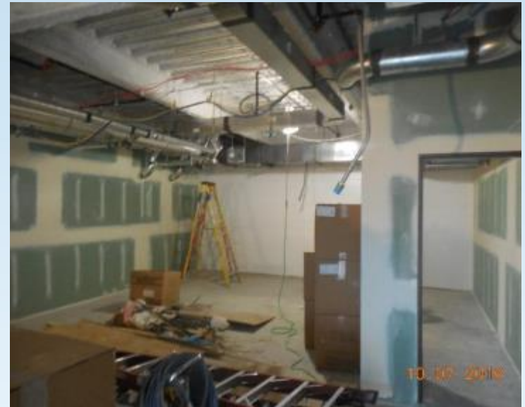
Kitchen Area in Progress
